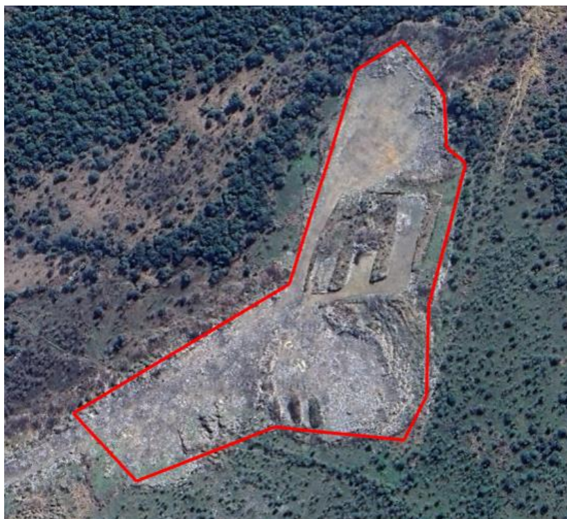
Figure 4-25: Alice Waste Disposal Site footprint
