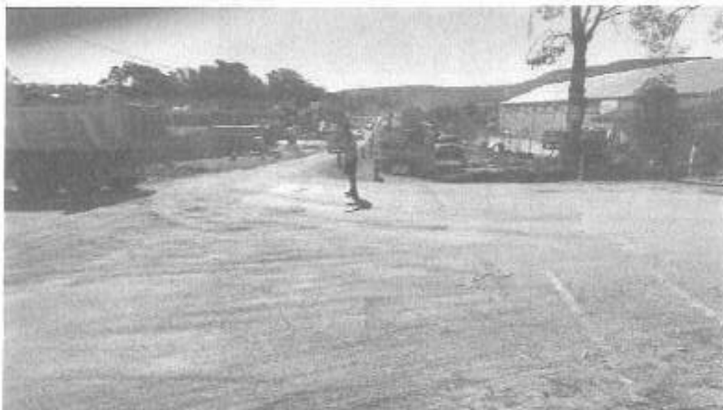
Grahamstown Road Box Cut and Widening
