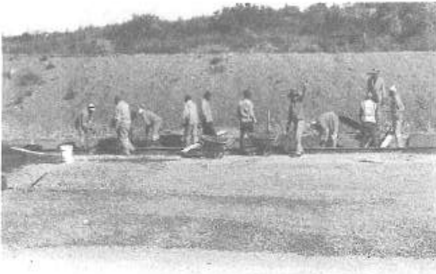
TE constructing Side Drains
