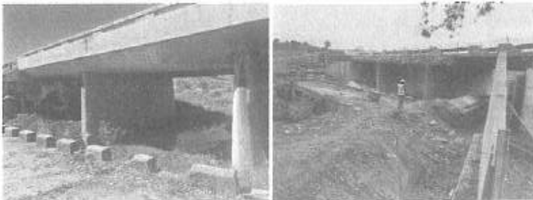
Brak River Widening: Before – Widening in Process
