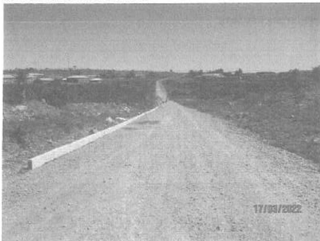
Photo 1: Kerbing on progress
