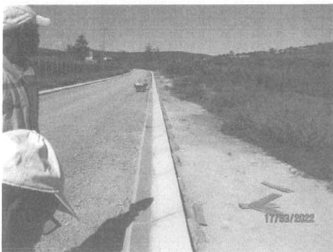
Photo 2: Kerbing and channel on progress
