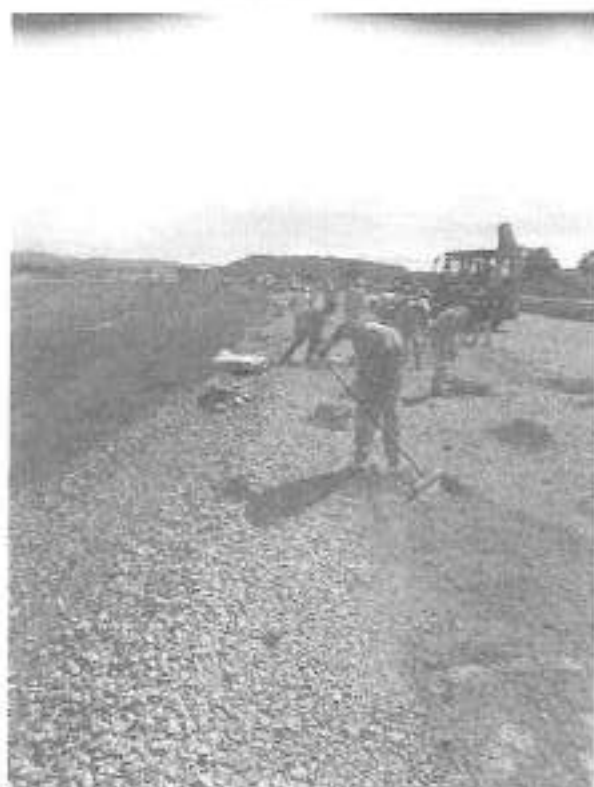
Stabilising subbase. TE's spreading cement
