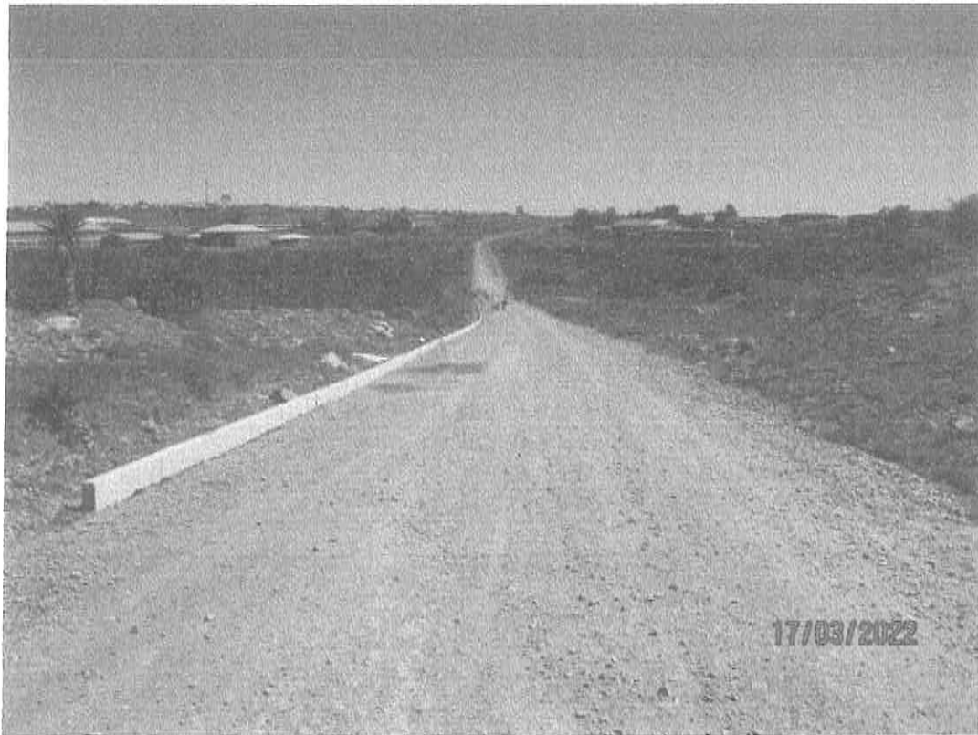
Photo 1: Kerbing on progress
