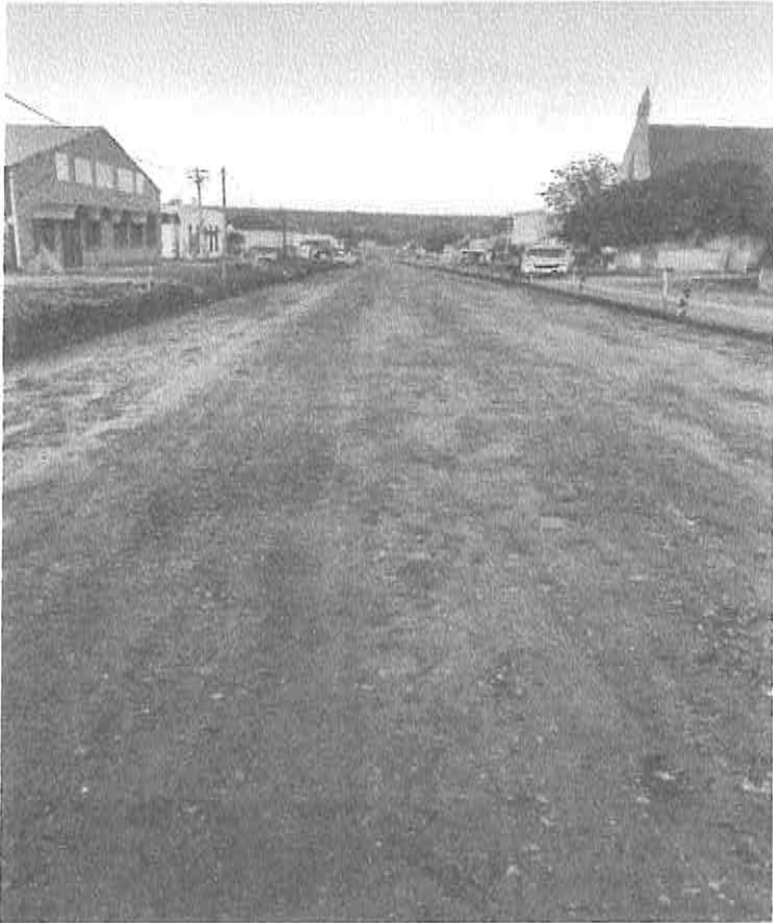
Campbell Street Box cut done. SSG Layer processed
