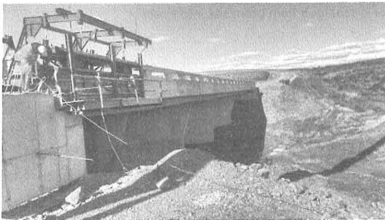
Mxelo River Bridge
