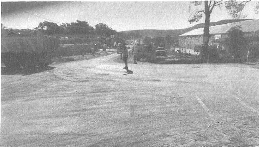
Grahamstown Road Box Cut and Widening
