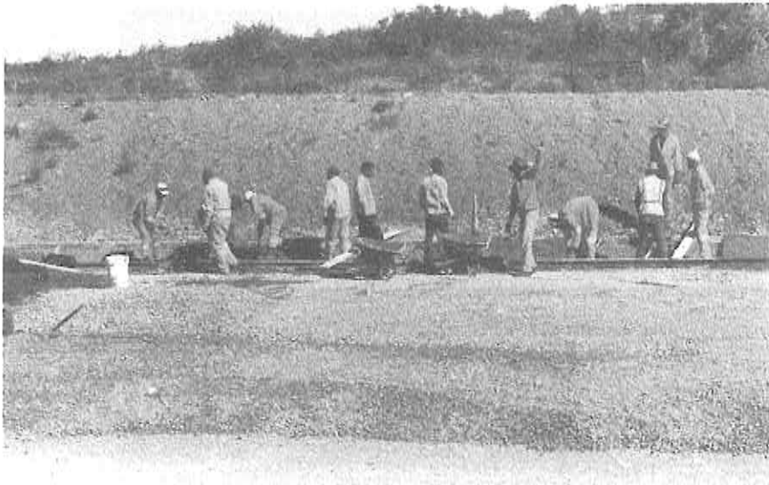
TE constructing Side Drains
