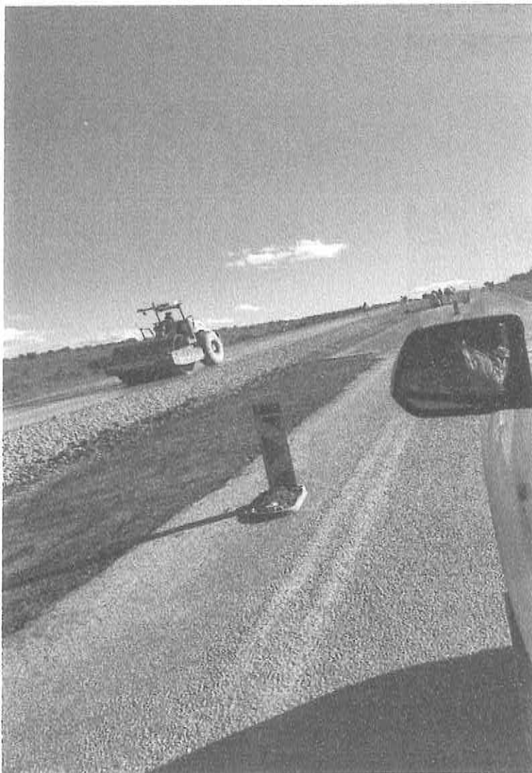
Base Patches on Bypass done by TE Contractor
