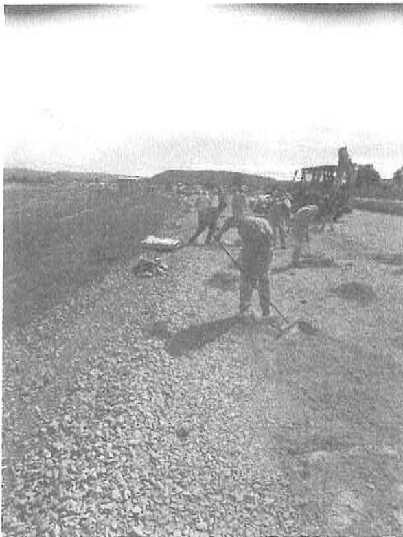
Stabilising subbase. TE's spreading cement
