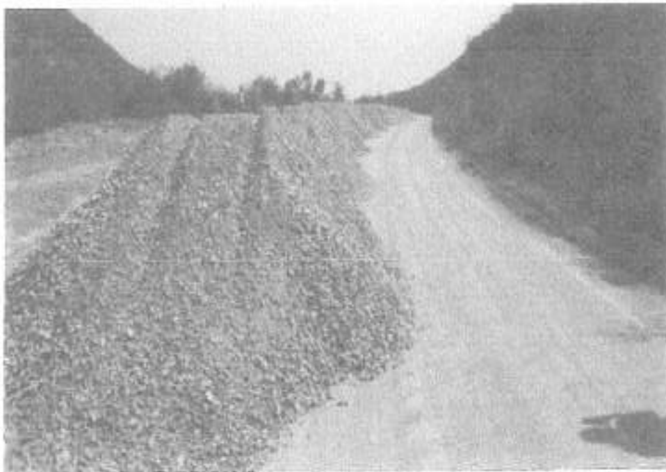
Photo 2: G5 material tipped
