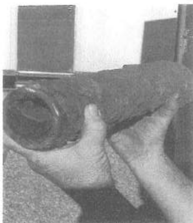
EXISTING BLOCKED WATER PIPES
