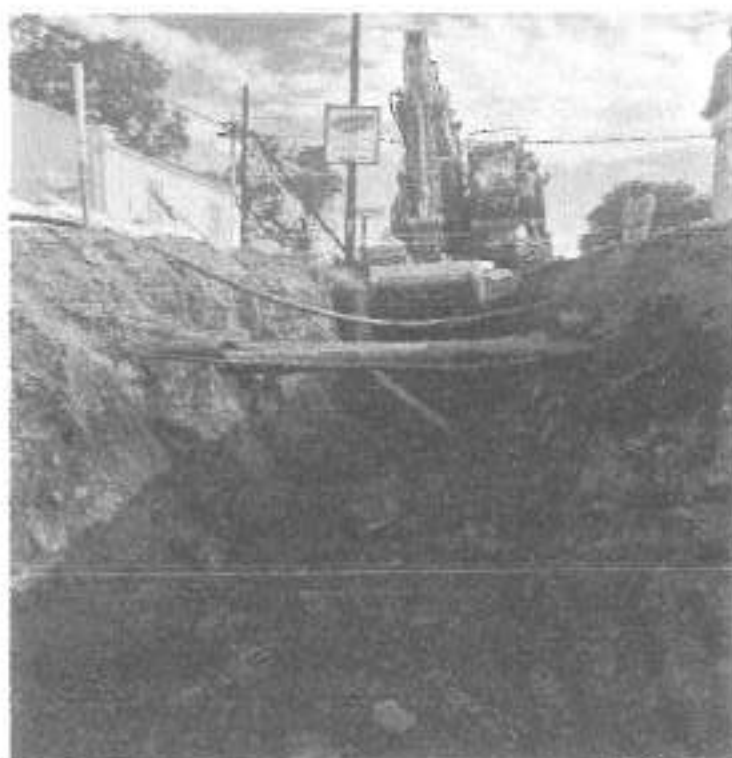
GRAHAMSTOWN ROAD: UNMARKED EXISTING SERVICES
