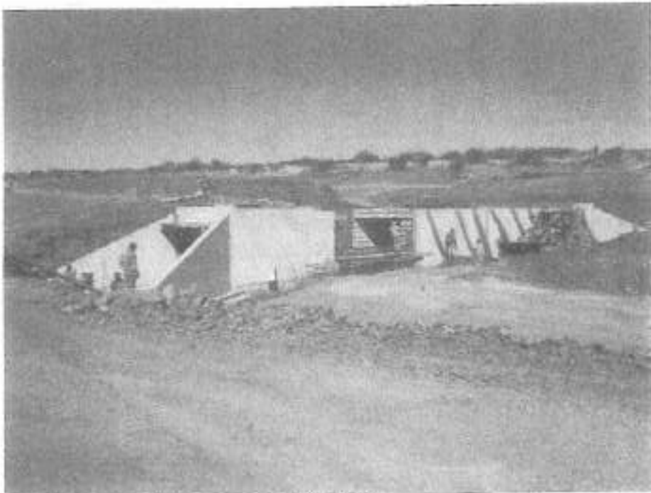
IN SITU CULVERT UNDER CONSTRUCTION
