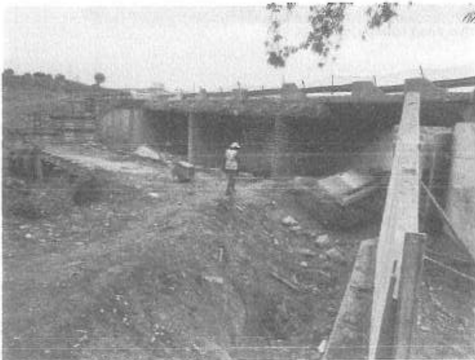
WIDENING OF BRAK RIVER BRIDGE LHS
