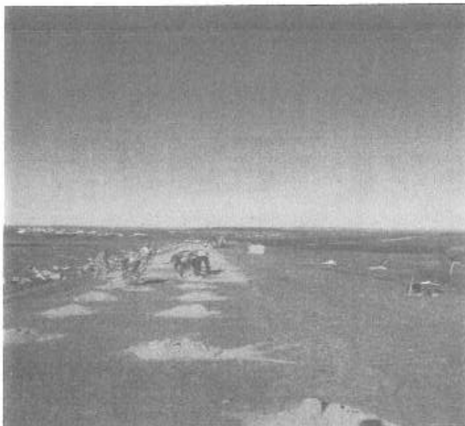
DISTRUBUTING THE CEMENT FOR SUBBASE STABILISATION
