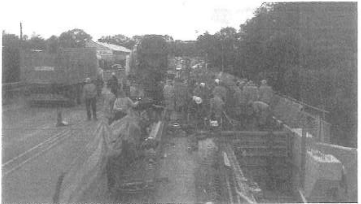
POURING CONCRETE ON KAT RIVER WIDENING RHS
