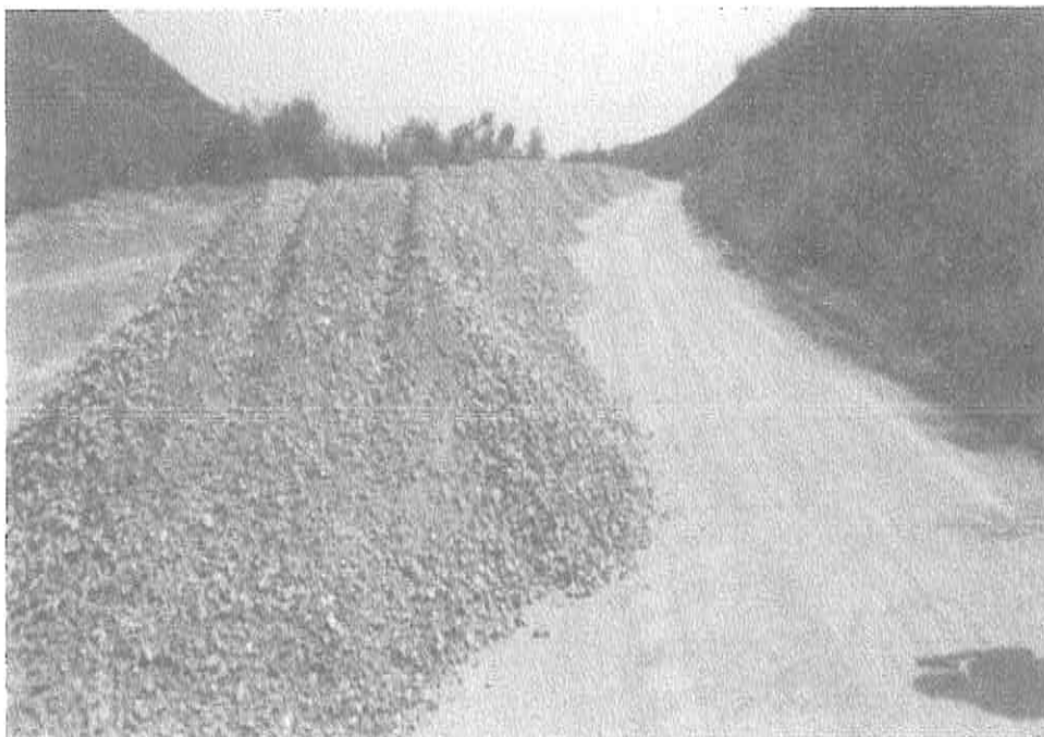
Photo 2: G5 material tipped
